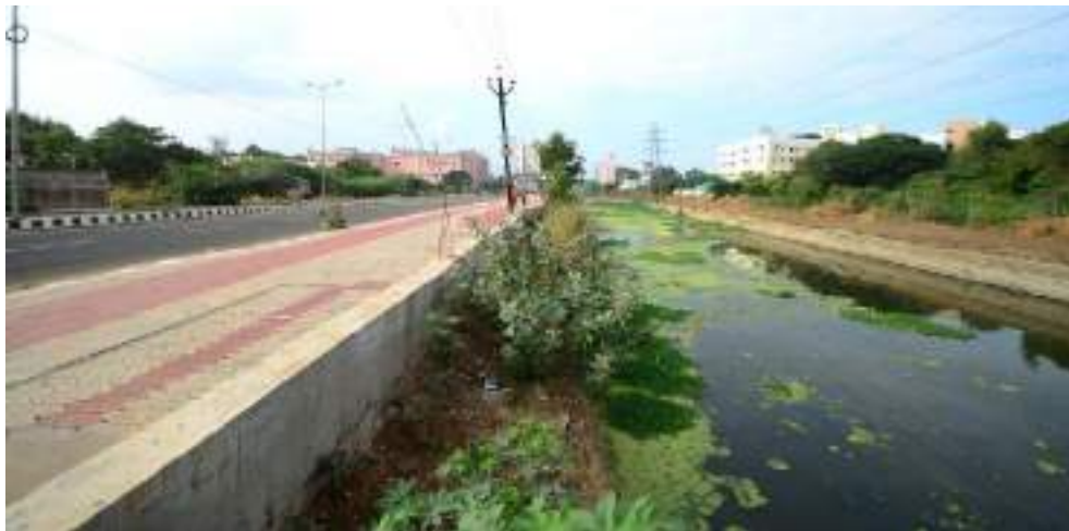
Figure 11-4 Absence Of Access Between The Banks
