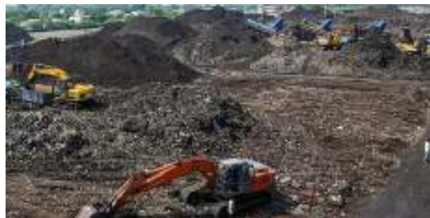
Figure 14-20: Existing situation of Ariyamangalam Dump Yard
