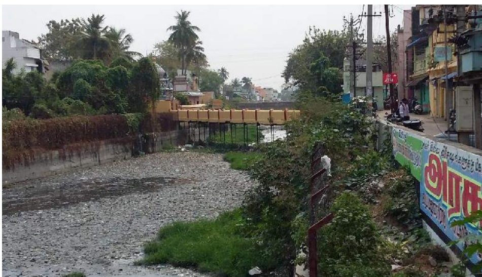
Figure 11-8 Improper Sewage And Solid Waste Management
