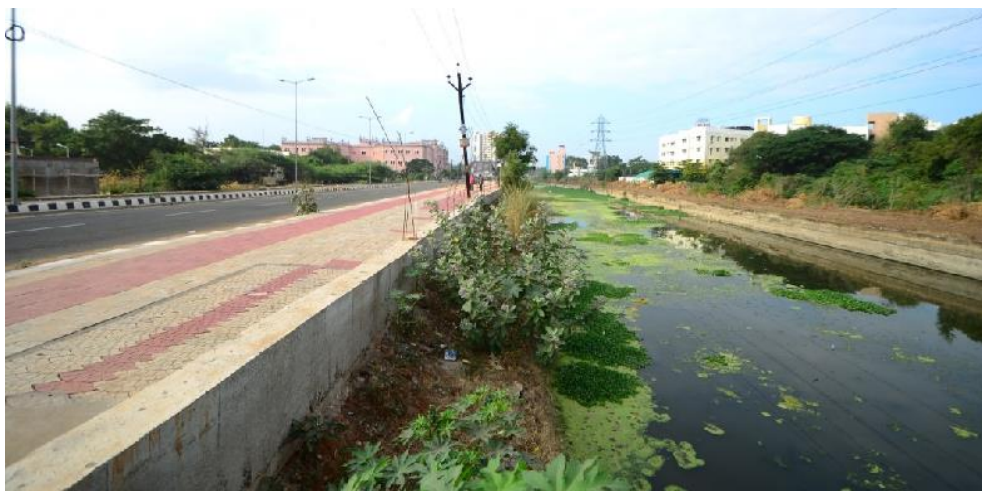
Figure 11-4 Absence Of Access Between The Banks
