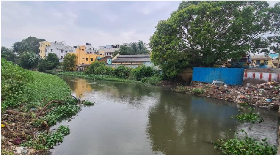
Figure 11-3 Illegal Occupancy/ Encroachments
